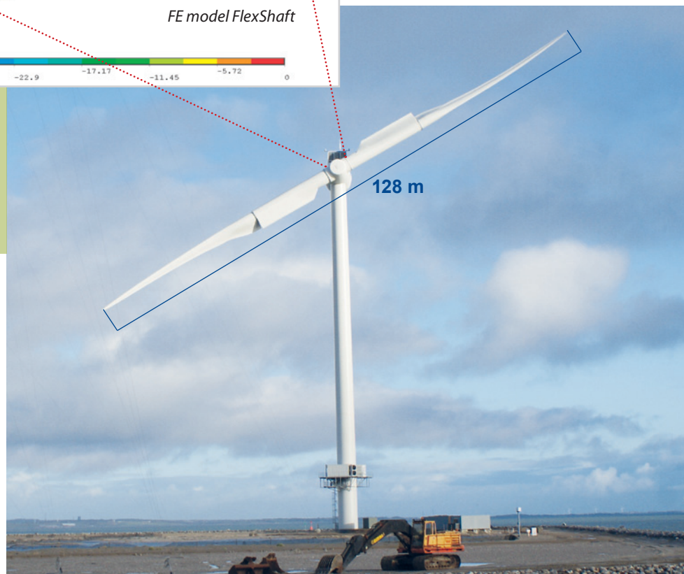
Windkraft-Anlage Wind energy plant
